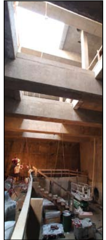
Tight working conditions and weather impacted complex pump station construction.
