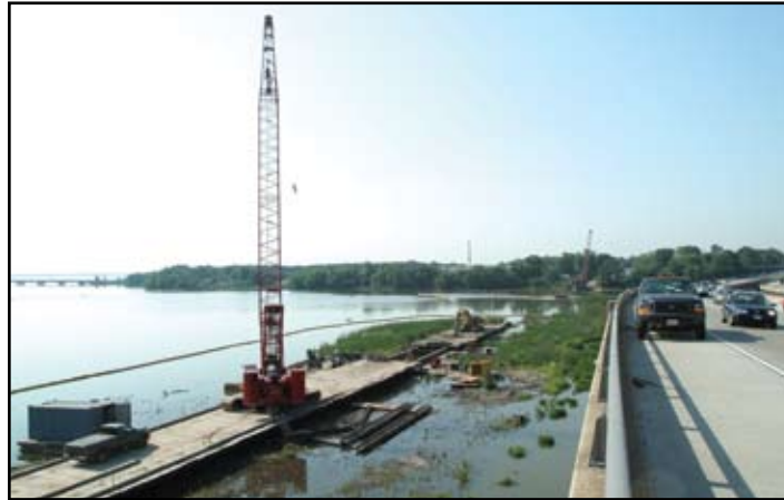
Temporary causeways facilitate installation of 54" force main fifteen feet below surface.
