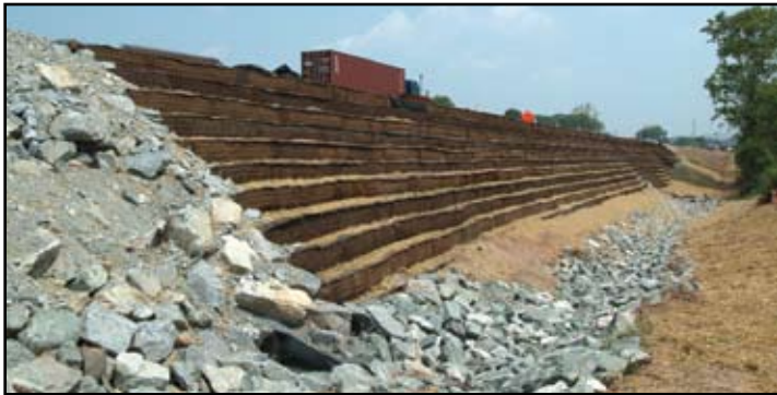
A reinforced soil slope (RSS) was needed to widen the Turnpike without encroaching on neighboring right-of-way. When complete, the steps will be hidden by fill, resulting in a constant slope.
