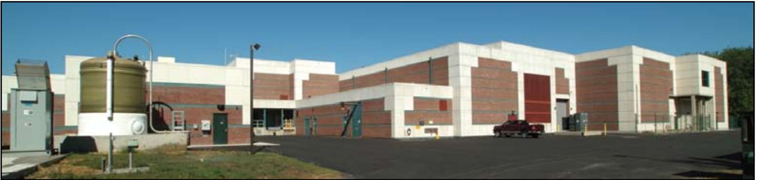
New chemical building and new GAC filter construction tie into existing construction.
