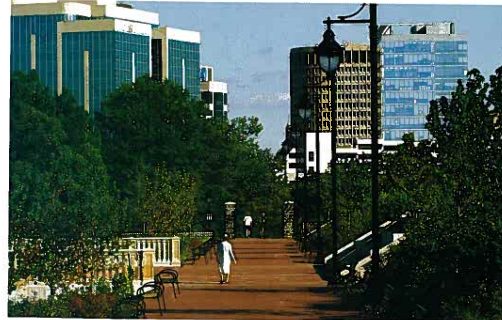
PARK LIFE The new Cool Spring reservoir occupies the south basin. On the north basin, pictured here, a park has been built, complete with a circular walking path, adequate lighting, benches, a field, and a pond. It opened to the public on Aug. 8. "There were a lot of hands in motion here," Cool Spring resident Sally O'Byrne says. "But you didn't hear or read anything negative about it, because there wasn't any controversy to speak of."
